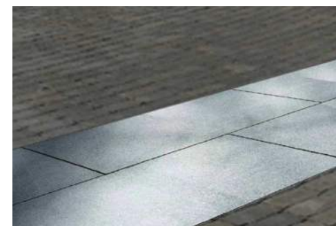
B 3' x 6' GRAY PRECAST CONCRETE PAVERS DESCRIPTION: PRECAST PANEL CONCRETE PAVERS COLOR: COLORED W/ CARBON POWDER FINISH: FINE HAIR BROOM FINISH SUPPLIER: PORTLAND CEMENT CONCRETE SIZE: 3' x 6' SCORING NOTES: DDOT STANDARD OR APPROVED EQUAL
