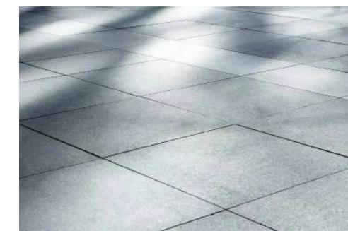
A 3' x 3' GRAY SCORED CONCRETE C.I.P. PAVEMENT TO MATCH R.O.W. IMPROVEMENTS DESCRIPTION: CAST-IN-PLACE CONCRETE COLOR: COLORED W/ CARBON POWDER FINISH: FINE HAIR BROOM FINISH SUPPLIER: PORTLAND CEMENT CONCRETE SIZE: 3' x 3' SCORING NOTES: DDOT STANDARD OR APPROVED EQUAL
